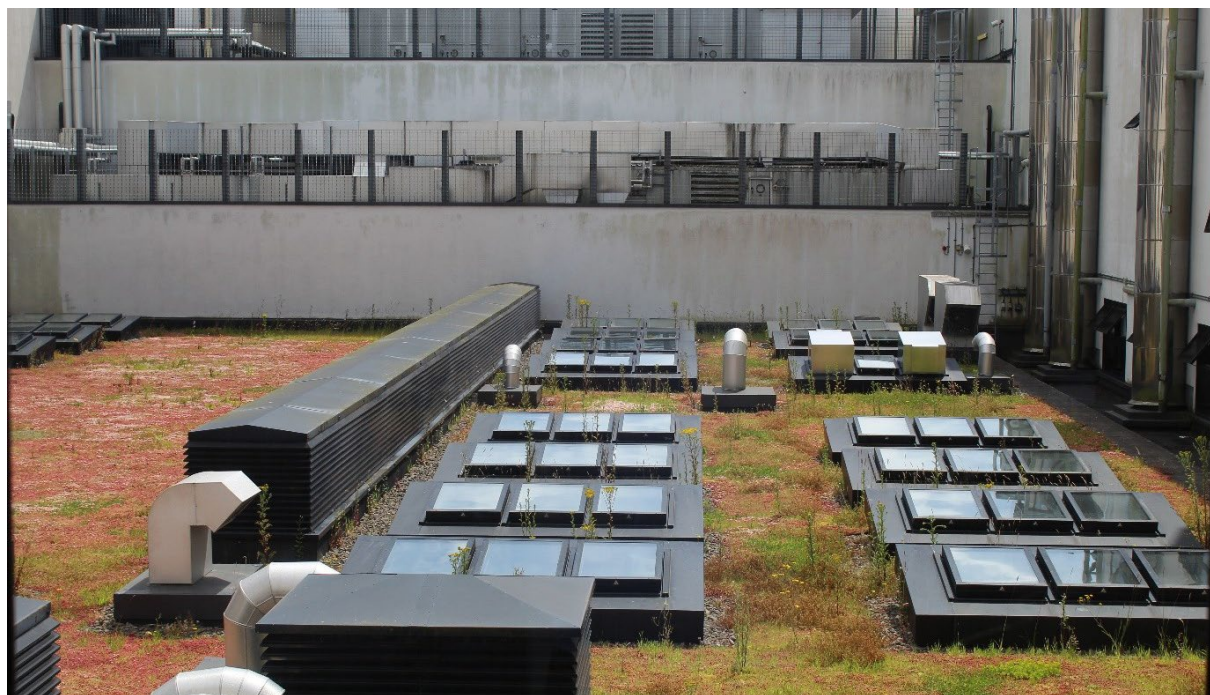
Figure 4.5 The Engineering Building's green roof
